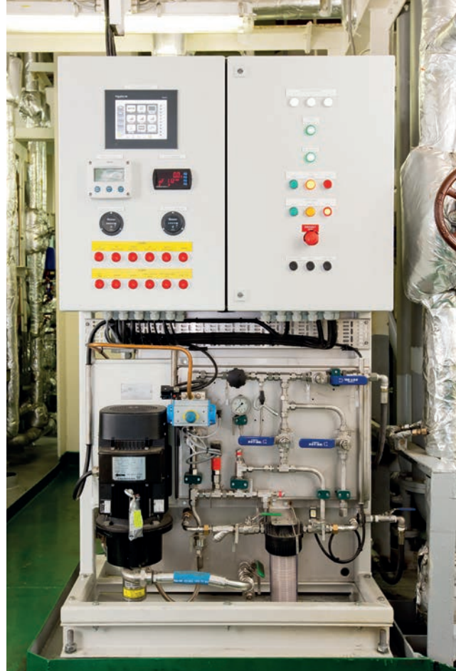
A water controller module of BOS emulsified fuel system.
