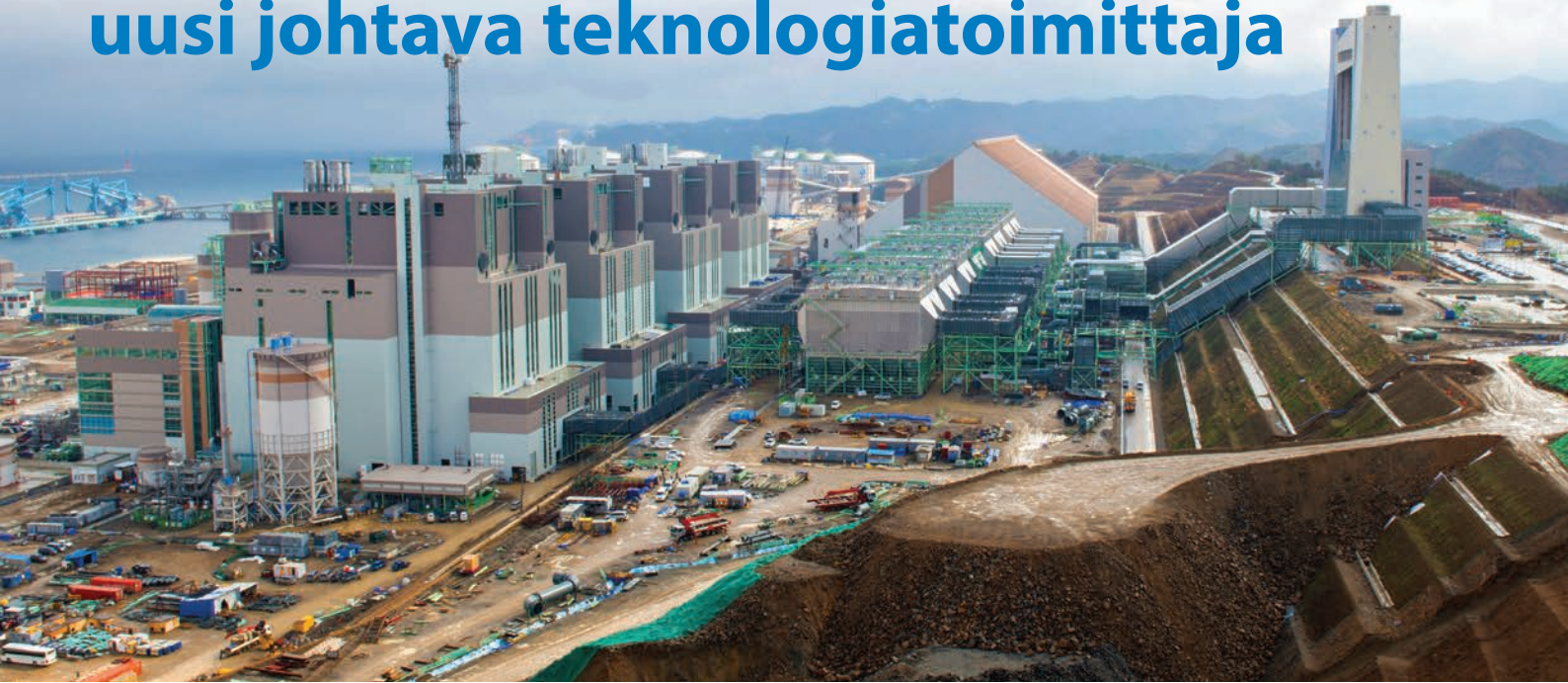
Samcheok Green Power Plant, Etelä-Korea, CFB 4 x 550 MWe.
