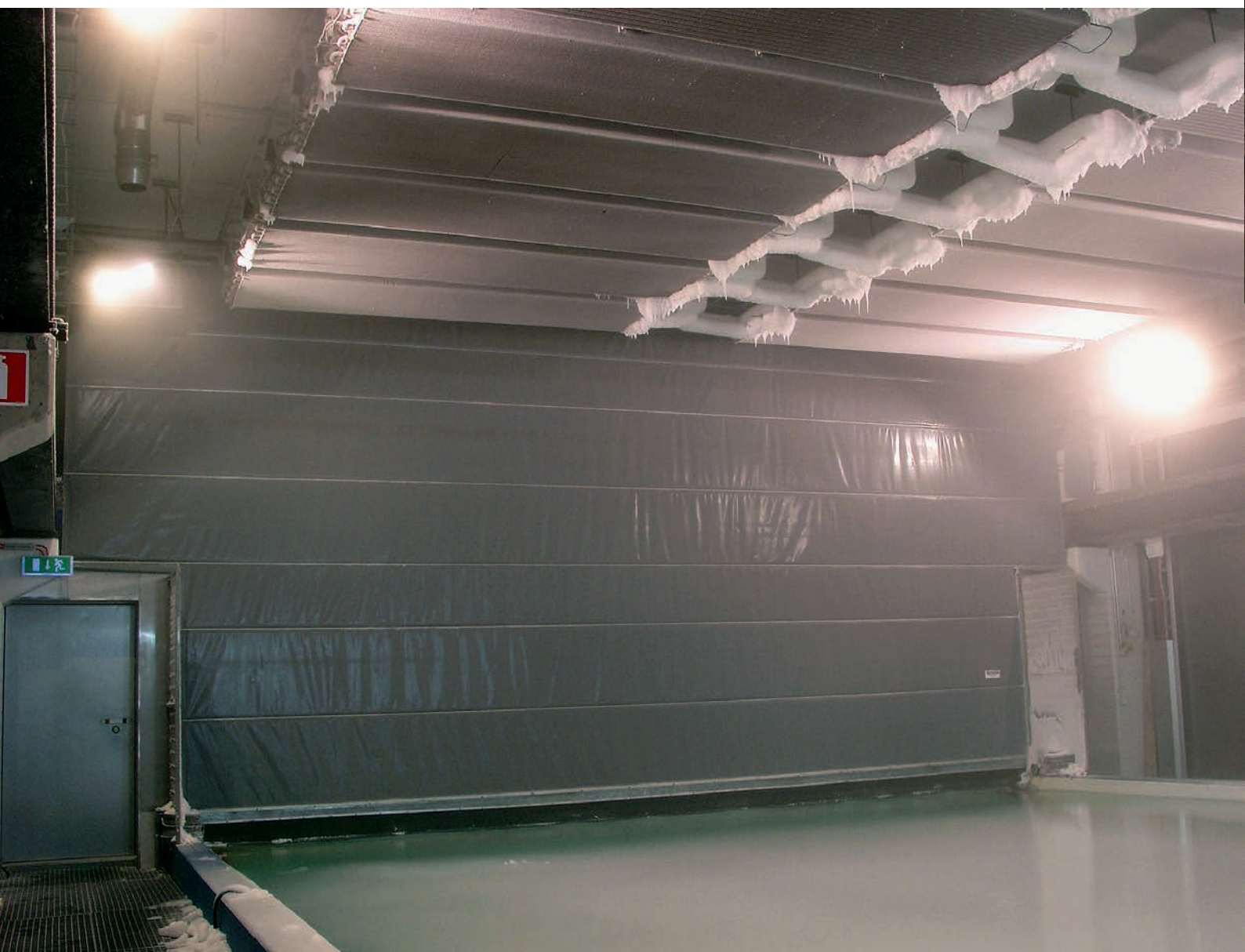
The NK4 Warm door installed for an ice laboratory in which solutions for the bow of the icebreaker are developed. The temperature on one side of the door is -20 C and +10 C on the other side.
