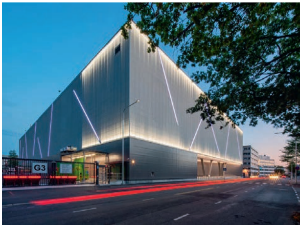
TELIA Helsinki Data Center, Helsinki
